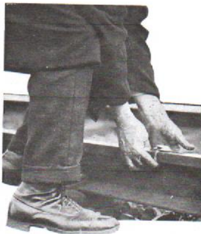
Clamping the warning detonator to the rail
