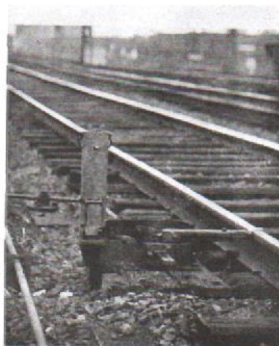
The Arm of a Clayton Fogging Machine Holding a Detonator on the Rail
