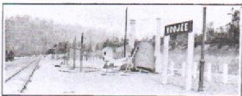
All that was left on the Noojee Station after the bush fires had passed through the district in February last. The remains of the gangers' and Stationmaster's residences are on the hill at the rear.
