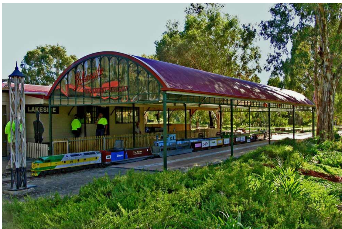
The delightful CVME Lakeside Station and Canopy awaiting some passengers.
