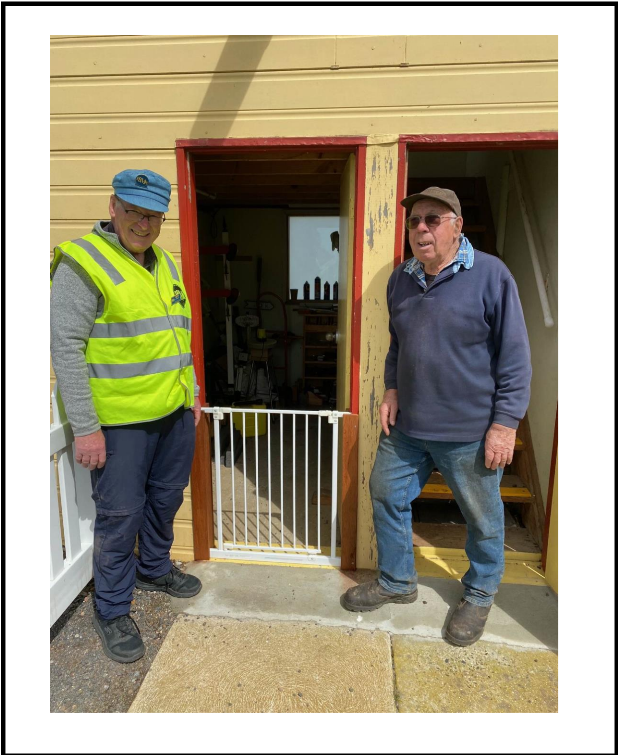
Keith Satterley (left) and Keith Stasinowsky (Right) admire the new security gate installed at the Point Richards Signal Box. They are two of our loyal volunteers whose efforts we much appreciate in keeping the “trains on the track”. (Pic: Brian Coleman)
