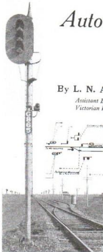
Style R., color light signal, the first of the type used in Victoria
